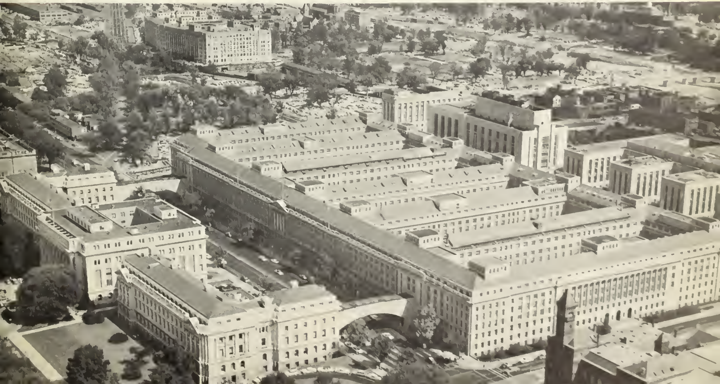
REA headquarters are located in the 2-block long South Building of the U.S. Department of Agriculture.
